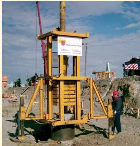
Dynamic load testing in the field
