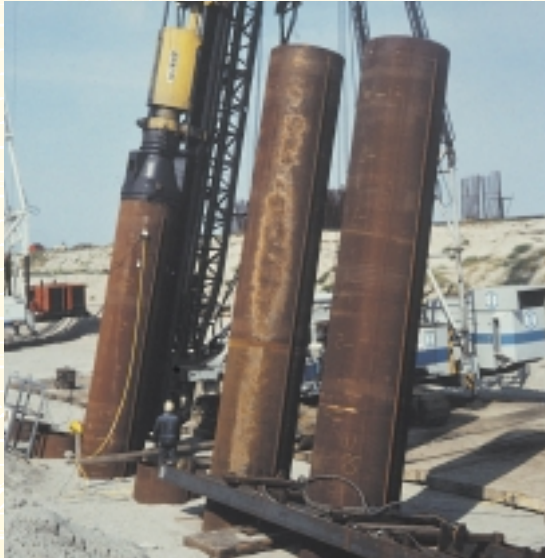
Pile monitoring with PDA.
