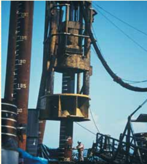
Pile driving monitoring offshore.
