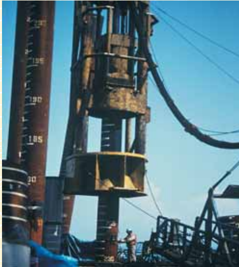
Pile driving monitoring offshore.
