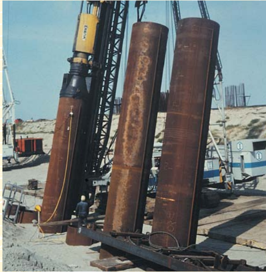
Pile monitoring with PDA.
